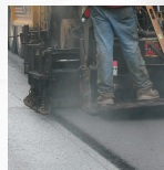
Mill and Overlay
