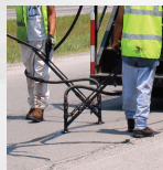
Crack Seal
