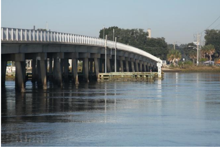
Bridge #2 2 Lanes Length 760' Width 39'
