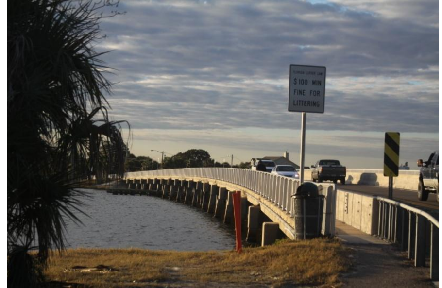
Bridge #3 2 Lanes Length 912' Width 35'
