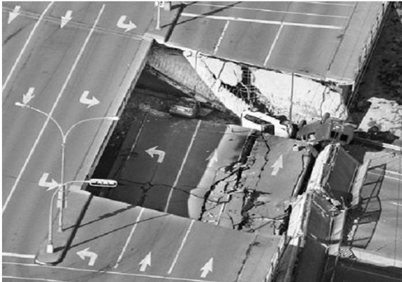
De la Concorde Overpass, September 30, 2006 Long-term deterioration caused collapse
