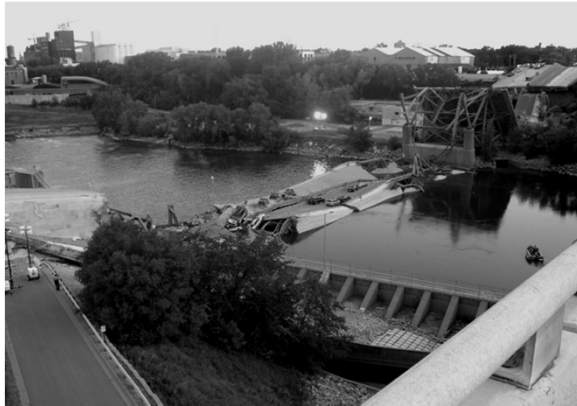
I-35W Bridge, August 1, 2007 Design error – under designed gusset plates
