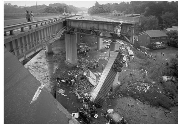
I-95 Overpass Collapse, June 28, 1983 Corrosion beneath pin hanger leads to fatigue
