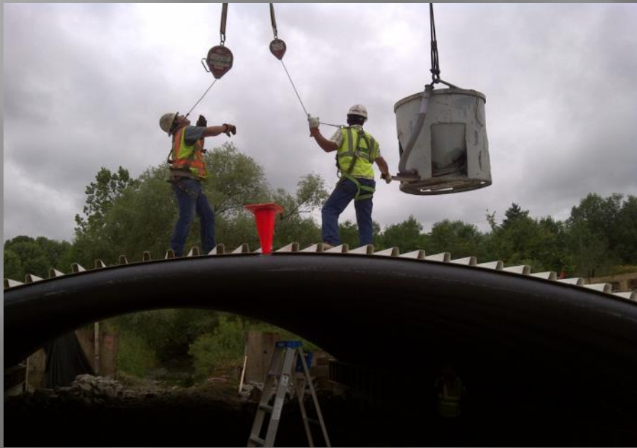
Pumping concrete into arches
