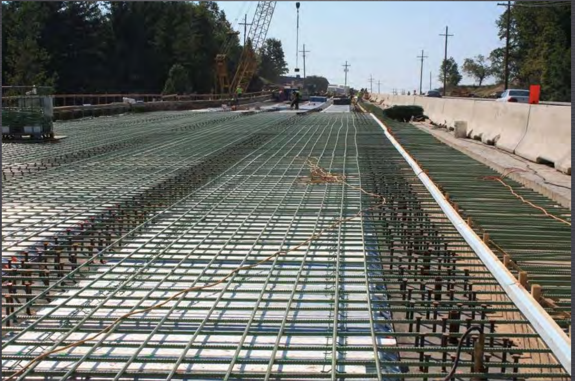
Deck Forms, Reinforcement and Shear Studs
