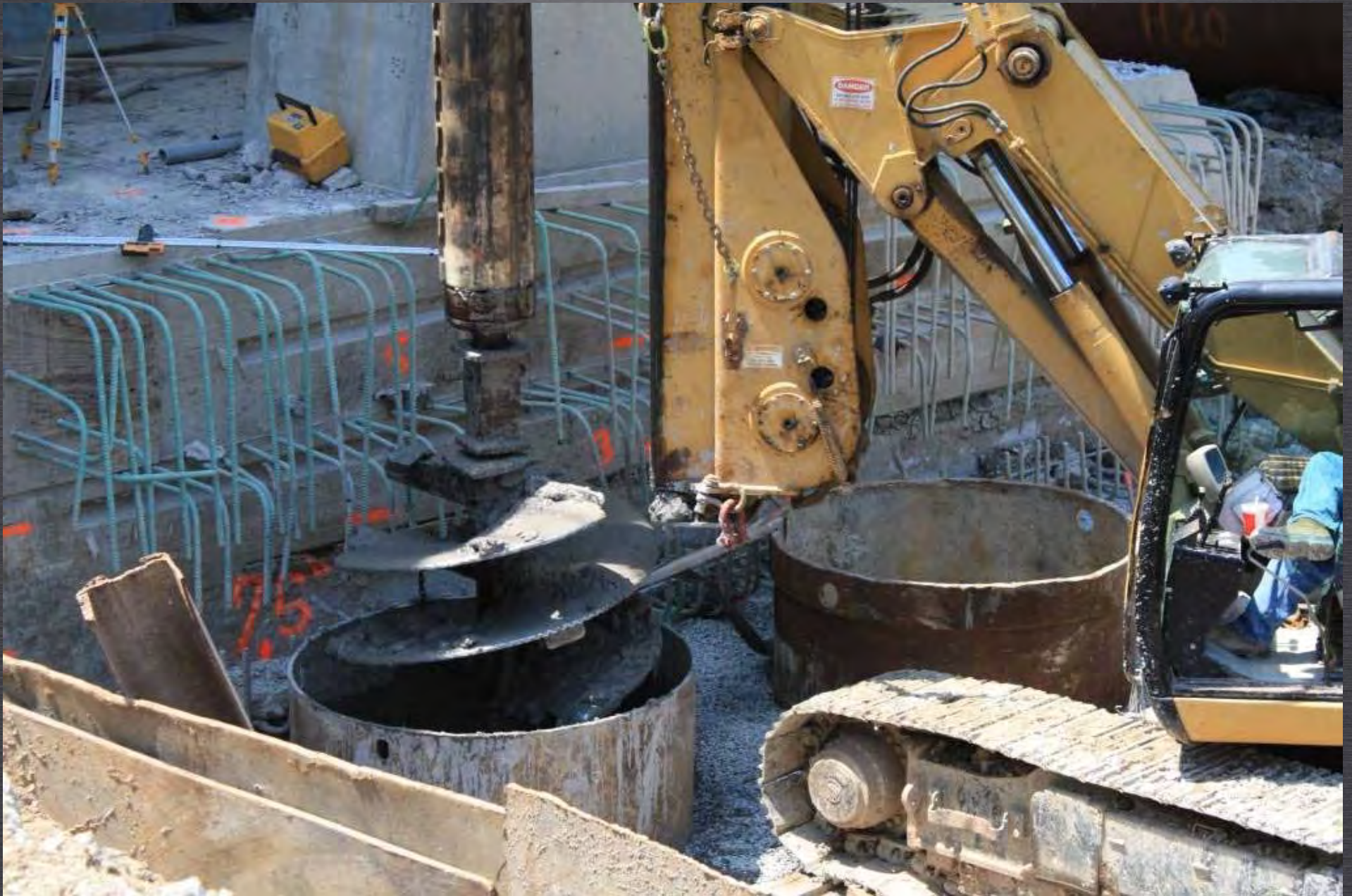
Drilled Shafts
