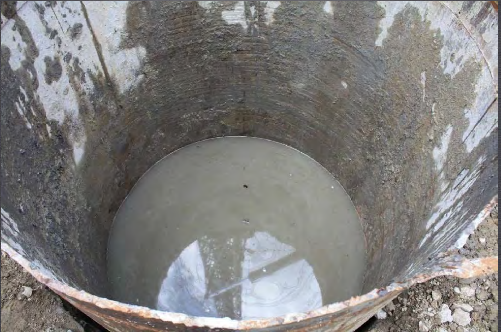
Drilled Shafts
