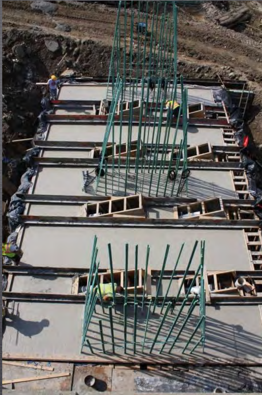
Pier Footing – Pour completed 12:30 pm
