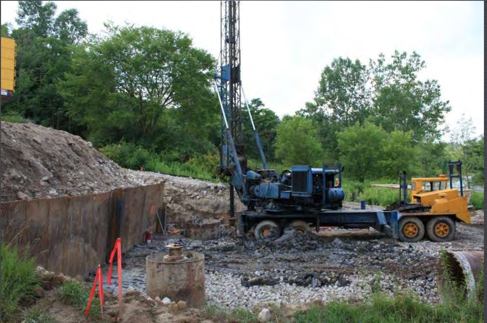
Drilled Shafts
