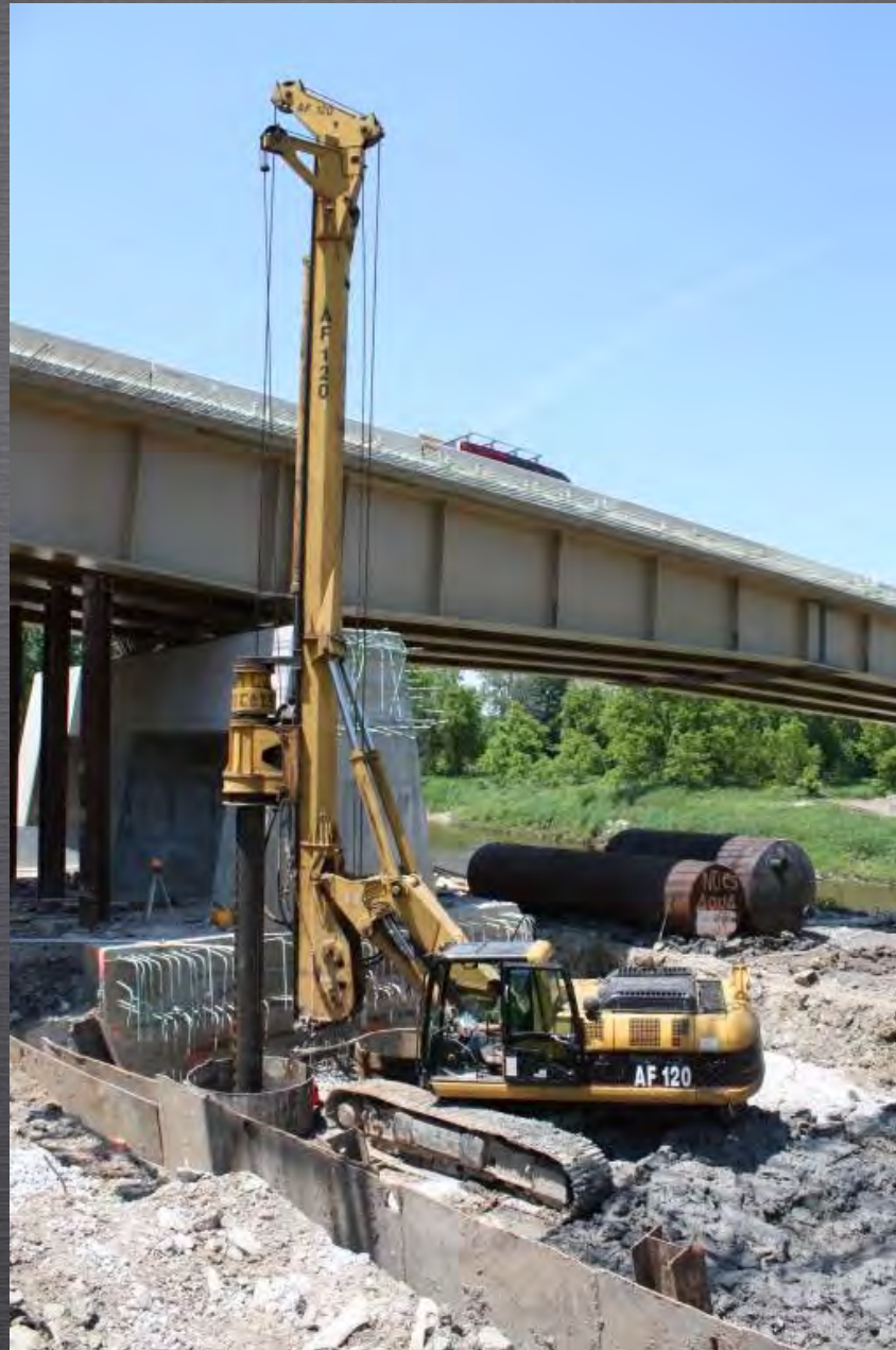
Drilled Shafts
