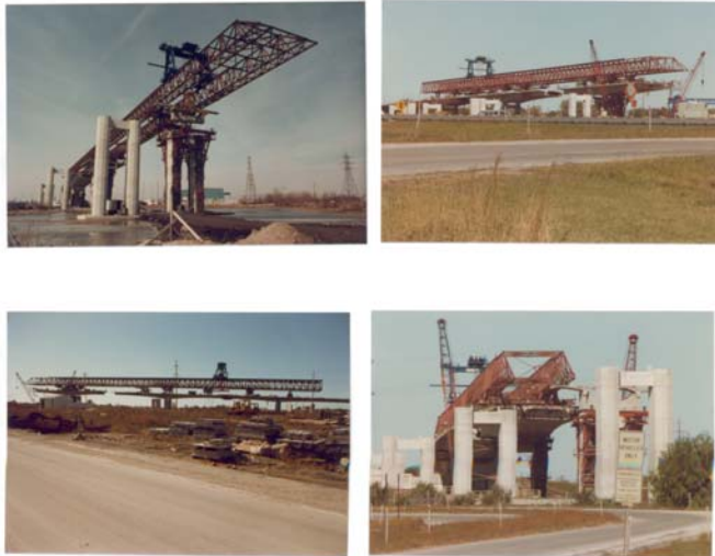
➤ Segment erection – launching girder
