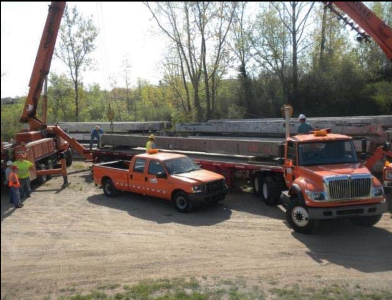
Salvaged box beam being loaded to be transported to LTU.
