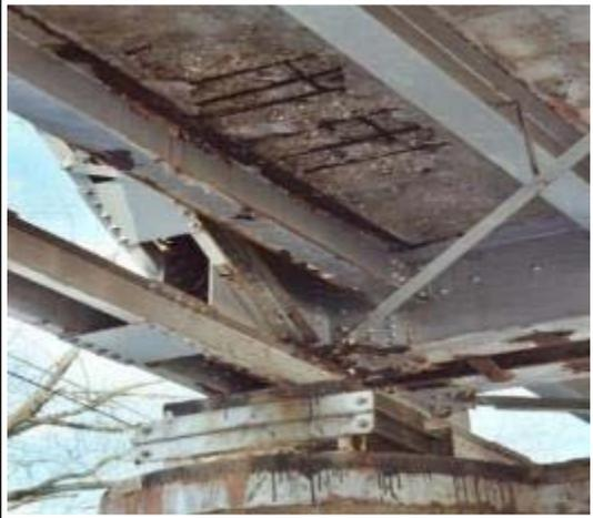
Corrosion of steel & concrete spalling
