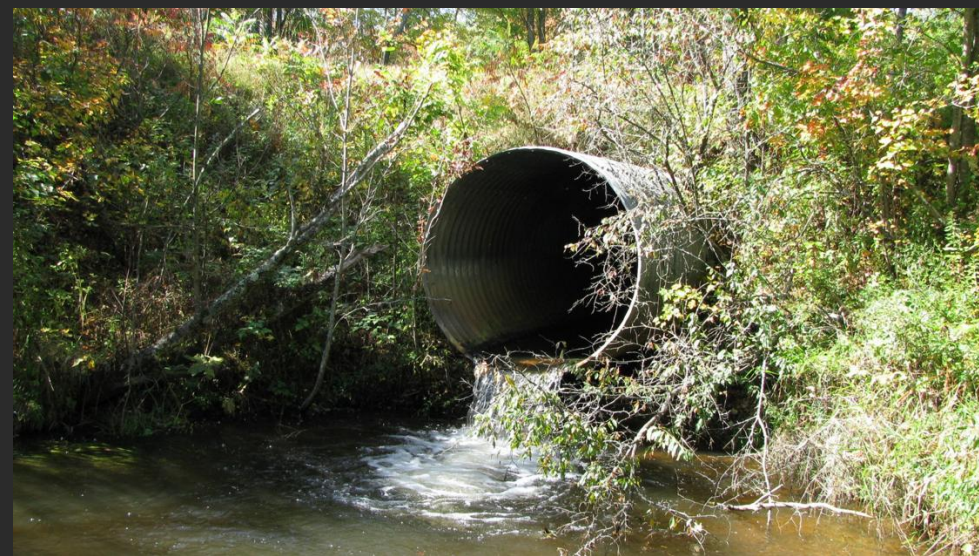
Perched Culvert above streambed
