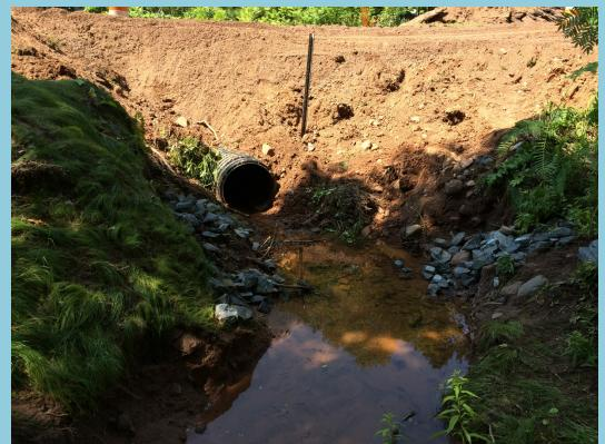
Putting in a structure with less waterway opening than what previously existed
