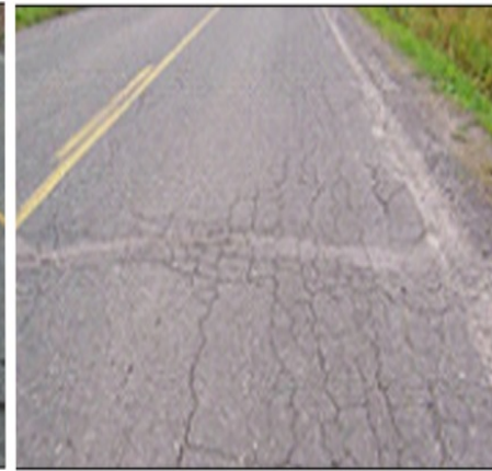
Alligator Cracking
