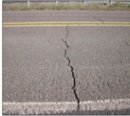
Transverse Cracking
