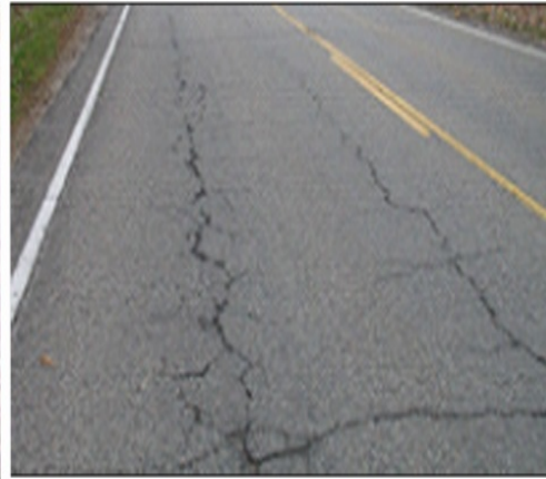
Cracking in the Wheel Path
