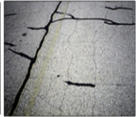
Block Cracking
