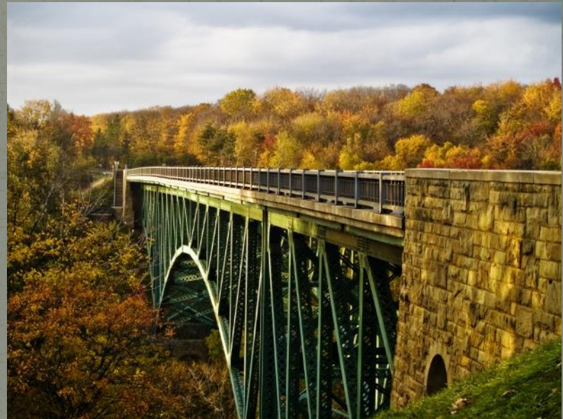
US-2 Cut River Bridge
