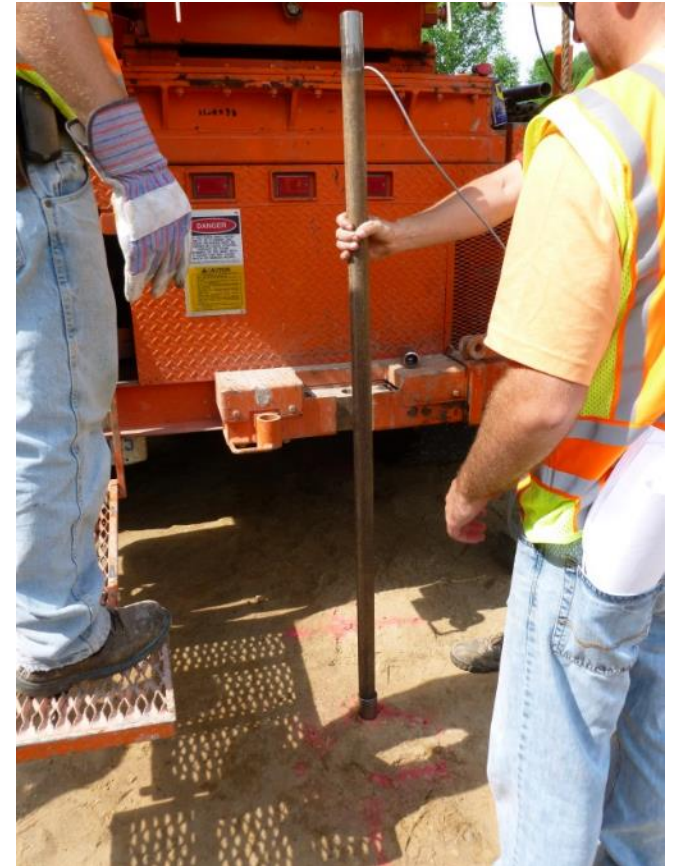
Installation of casing
