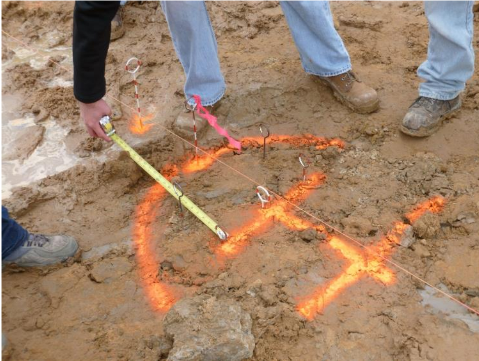
Positions for sensor installation
