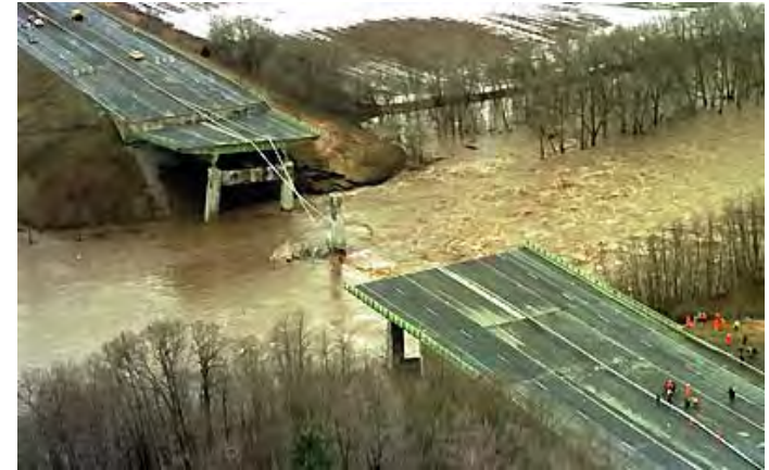
Thruway Bridge: Scour failure, New York. (Source: Associated Press, 1987)
