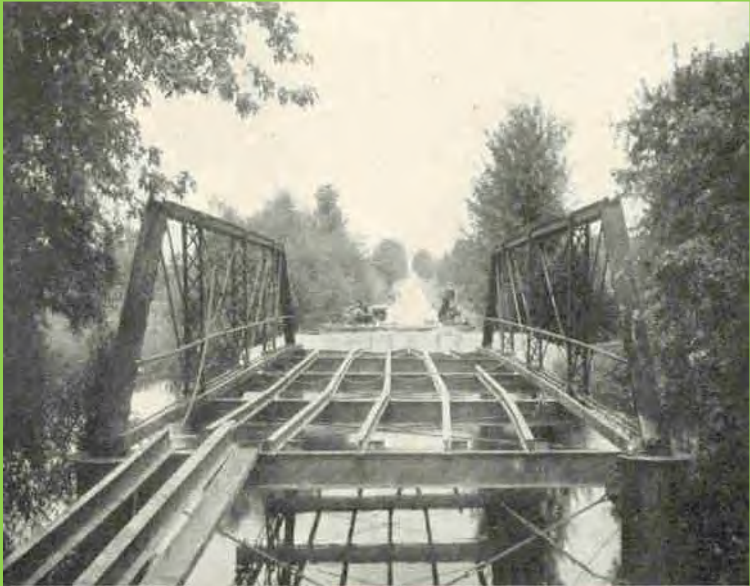
Original truss bridge being removed in 1925
