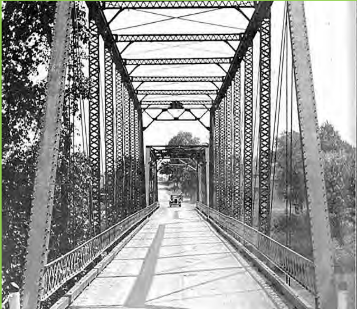
Typical 1920's truss bridge
