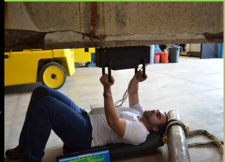
Scanning on Corroded Strands
