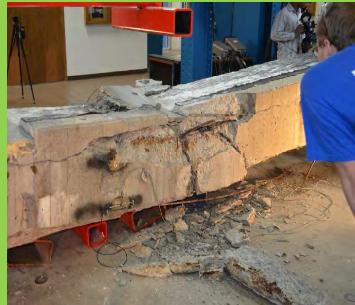
Salvaged Beam #1 (J11)
