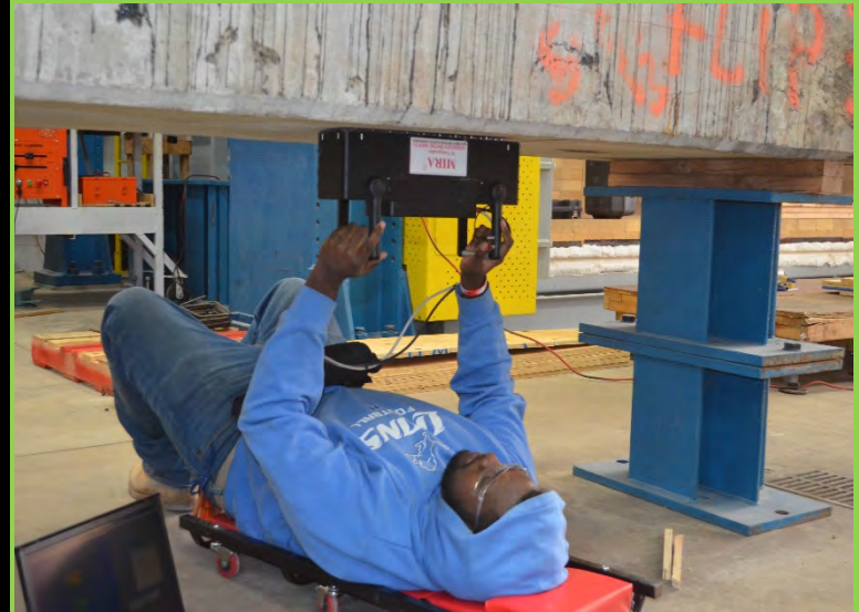
Scanning on Less Corroded Strand
