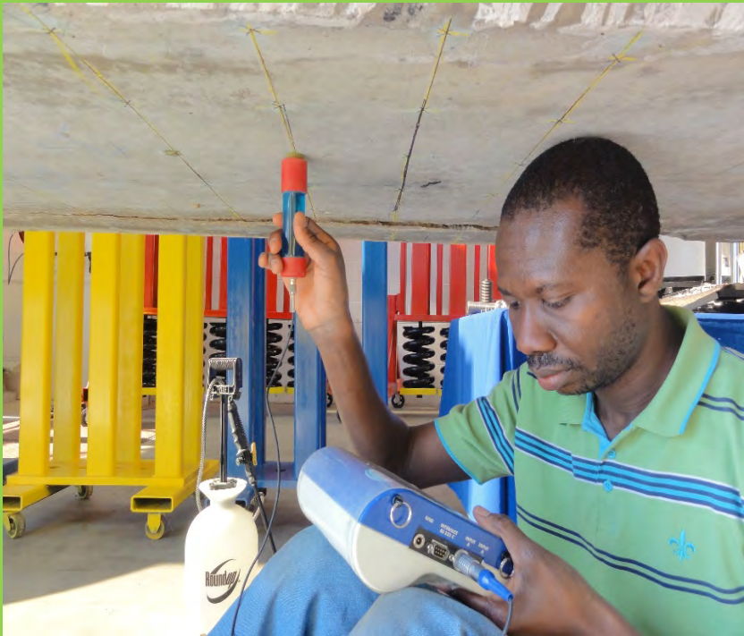
Half-cell potential measurement of bottom strands
