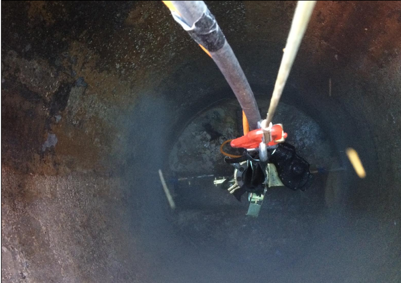
Manhole Being Coated
