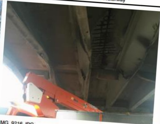
IMG_9216.JPG Beams 1-4s are shown, looking roughly west along Span 3w. Note condition of diaphragm attachments to angles.
