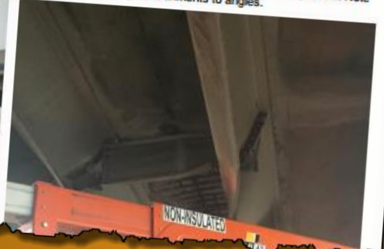
IMG_9216.JPG Beams 1-4s are shown, looking roughly west along Span 3w. Note condition of diaphragm attachments to angles.
