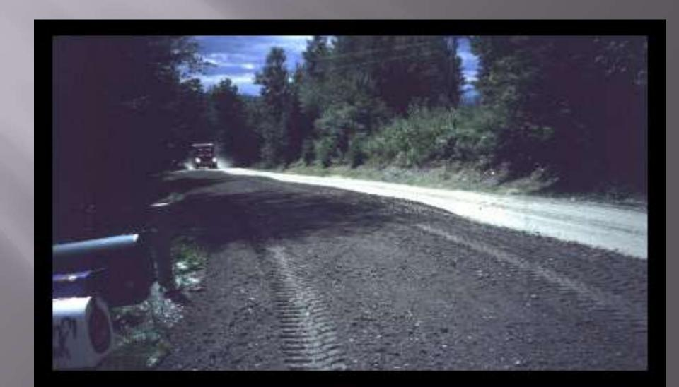
2 YEAR STUDY: PLACED 500 TONS OF RAS (GROUND TO LESS THAN 1". MATERIAL WAS GRADED BACK & FORTH TO MIX WITH GRAVEL. RESULTS INDICATED MUCH REDUCED DUST CONTROL NEEDS, LESS RUTTING AND LESS GRAVEL LOSS.
