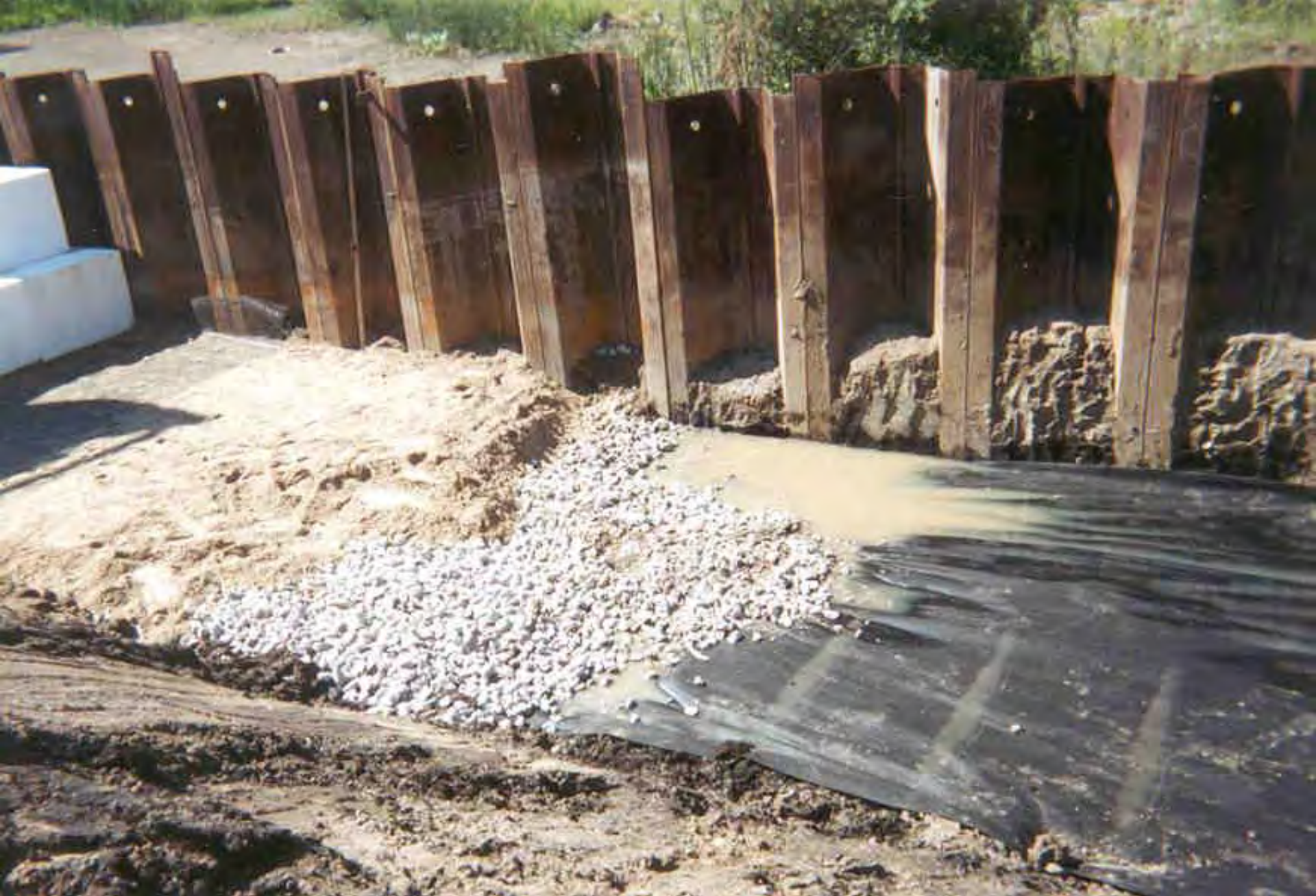
Preparation of marsh surface at base of EPS
