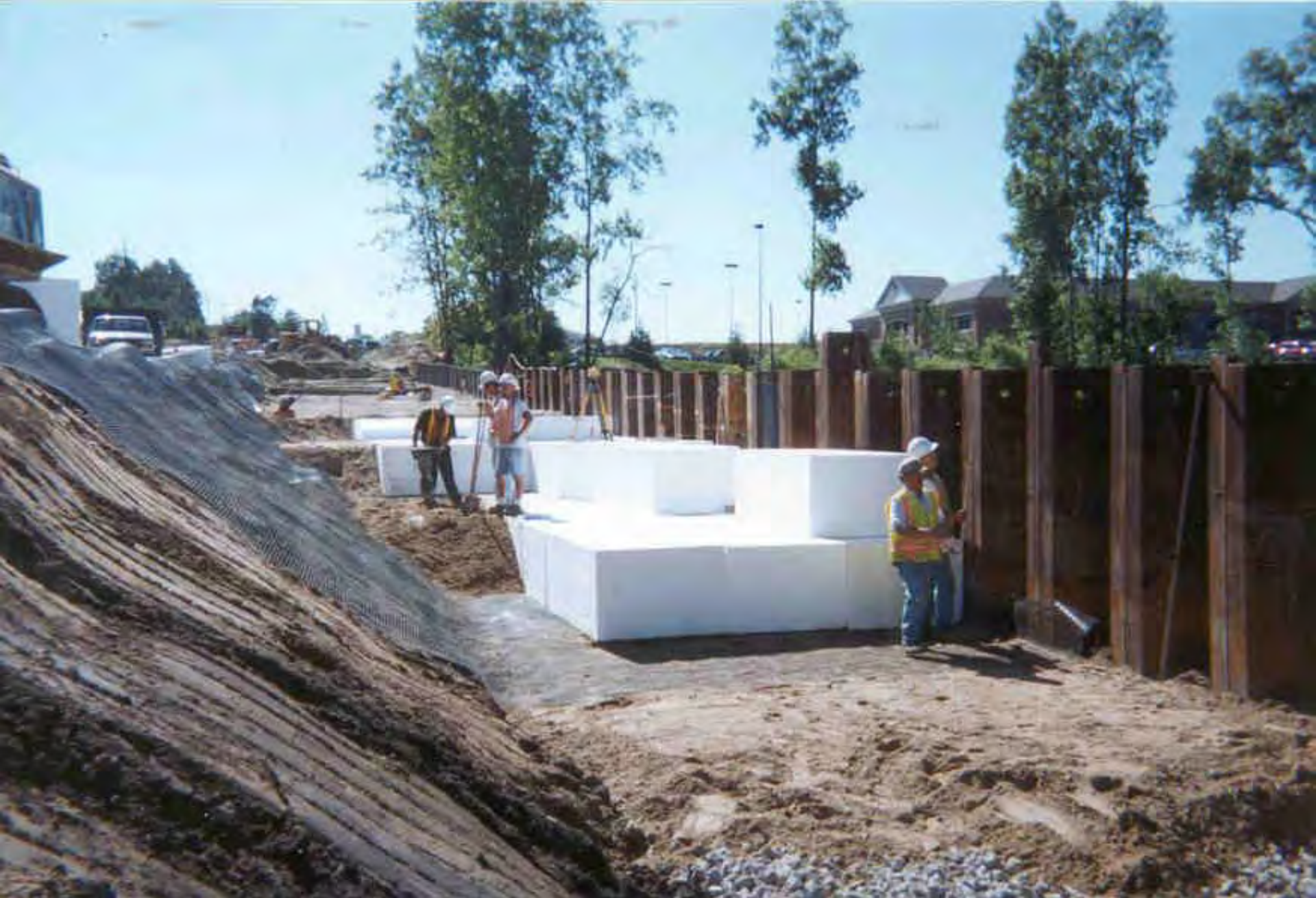
Placement of EPS and Geogrid behind sheeting.
