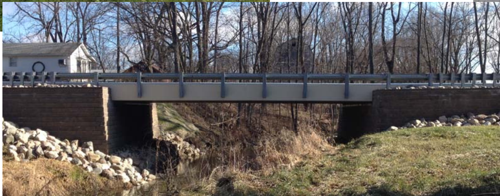
Kefer Highway over Sebewa Creek
