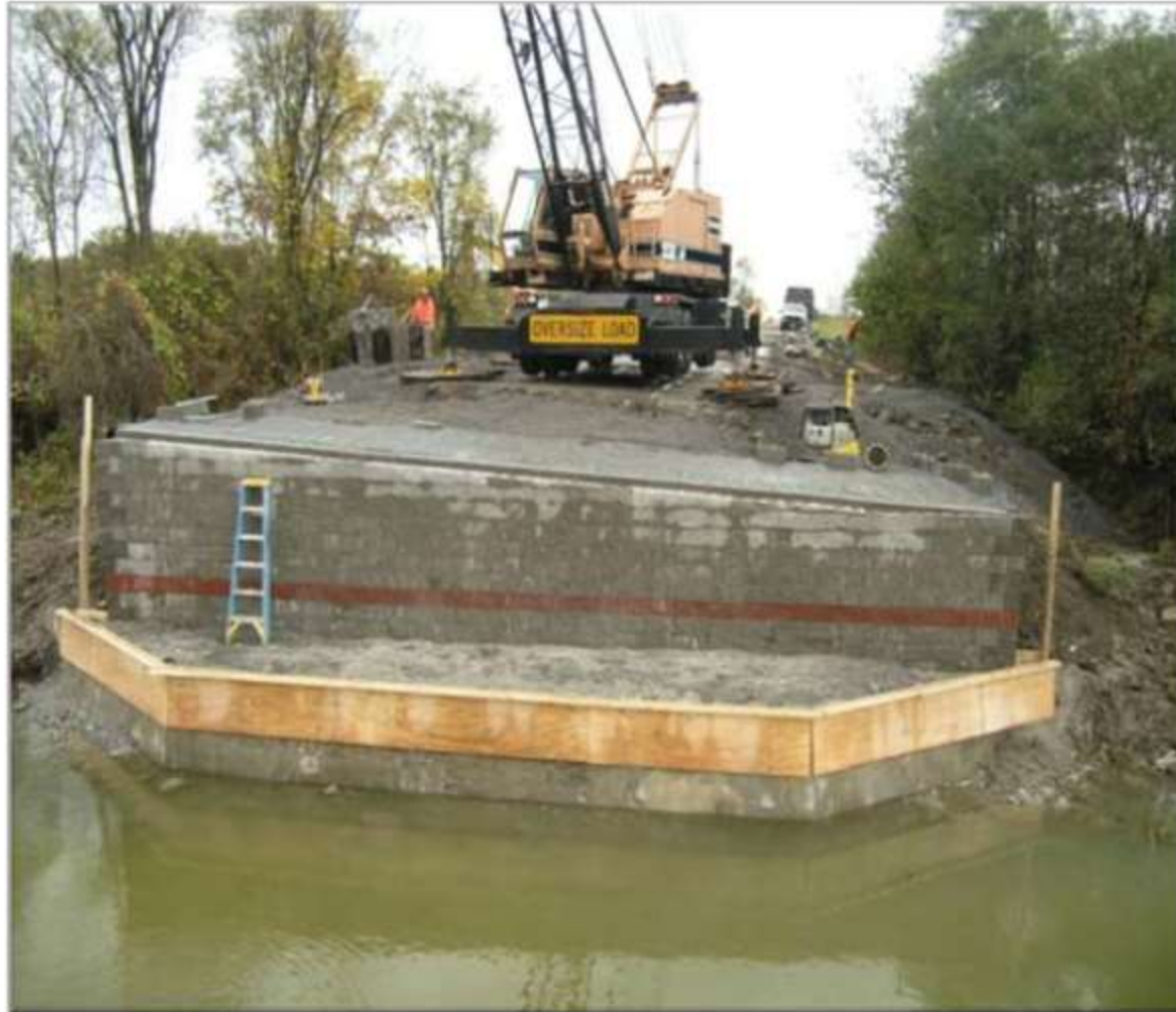
Figure 43. Photo. GRS-IBS built behind an existing concrete abutment.
