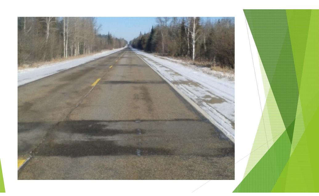
Widen for safety Add 4' paved shoulders Repair joints (details 7's) Test joints constructed (12) Mill to remove ½" ruts Resurface with high volume Ultra-thin pavement Maintain cracks over time
