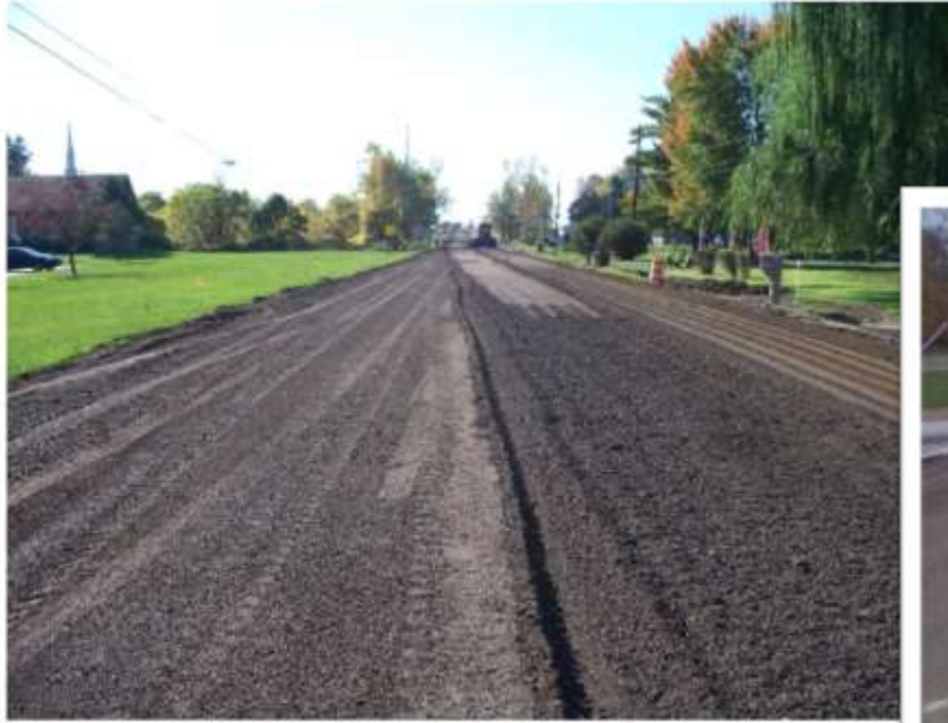
Grading Stabilized Base
