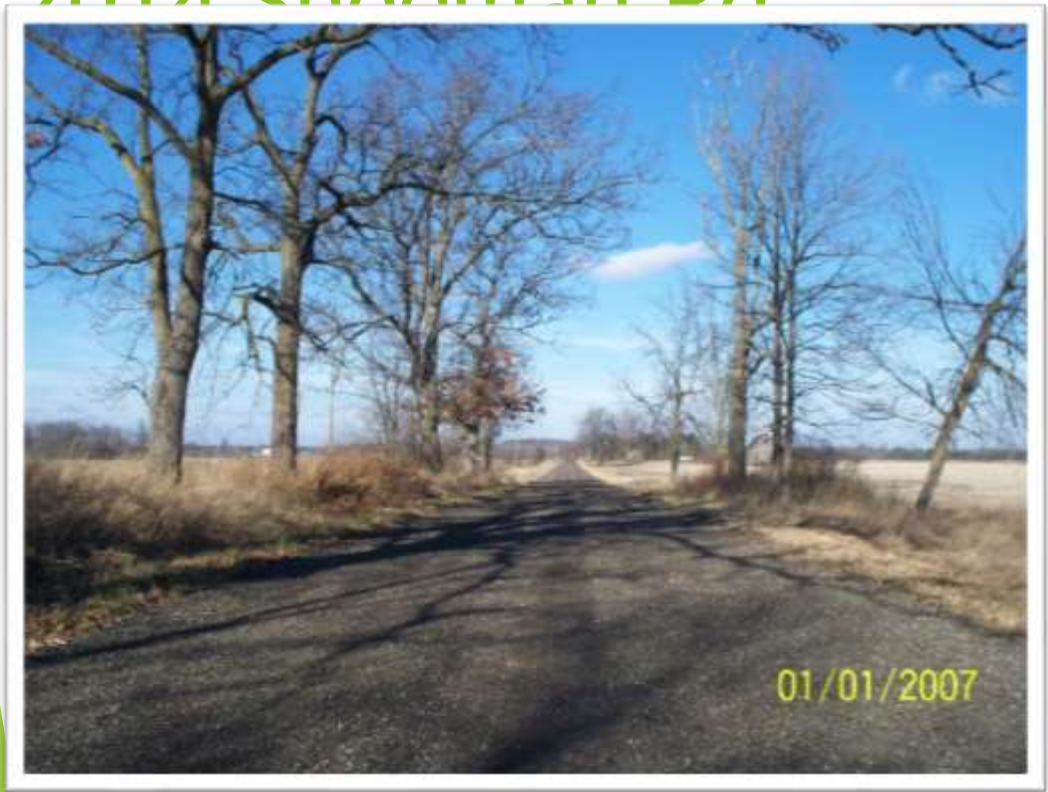
RAP Surfaced Local Road
