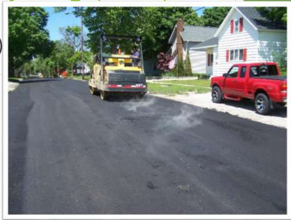
Compacted HIPR Surface
