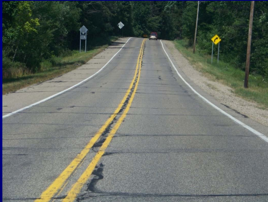
M-21, Before Construction
