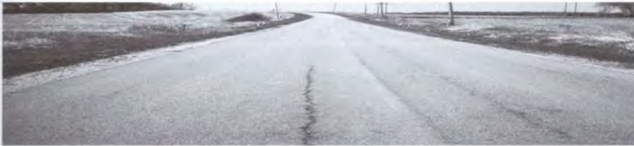
➤ Longitudinal cracking; early load-related distress in wheel path. Strengthening needed.
