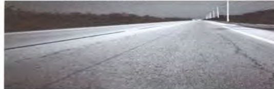
Load cracking and slight ▼ rutting in wheel path.
