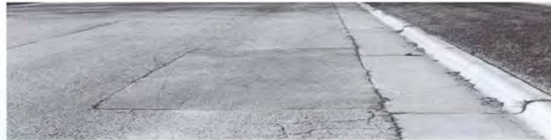
➤ Extensive block cracking. Blocks tight and sound. ➤ Slight rutting in wheel path.
