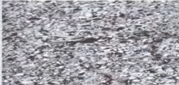
Severe raveling with ▼ extreme loss of aggregate.
