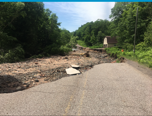
In 2018, a catastrophic rain event caused severe damage to Houghton County Roads. Kevin Harju will present on the recovery effort and what can be expected when working with other agencies.
