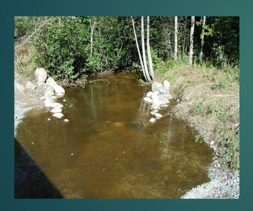
Use cross vanes as grade control to permanently set a channel invert
