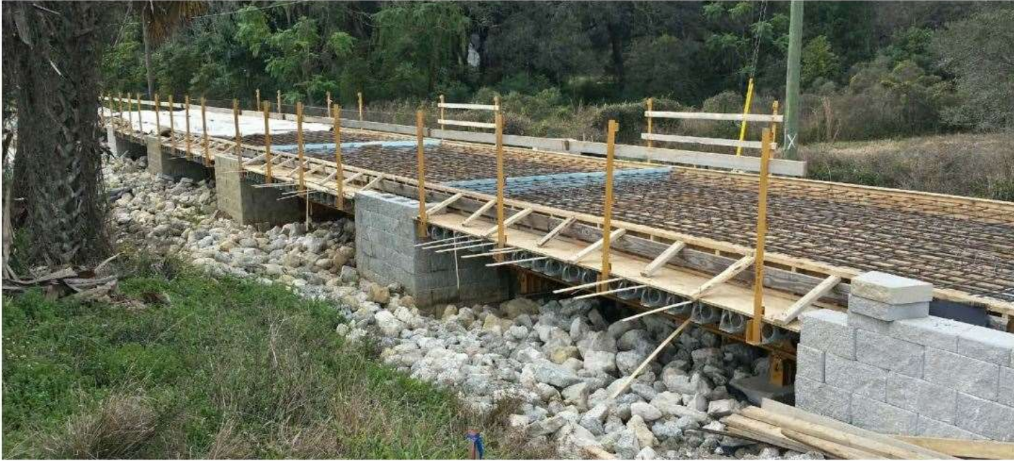
Figure 3. Construction of U.S. 301 Trail Bridge with multi-span GRS-IBS in Zephyrhills, Florida.
