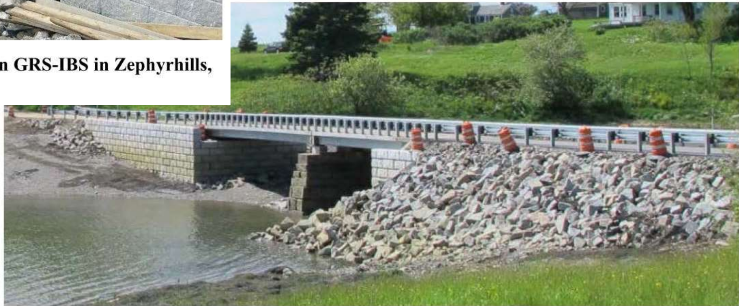
Figure 4. Completed two-span GRS-IBS bridge in Knox County Beach, Maine.
