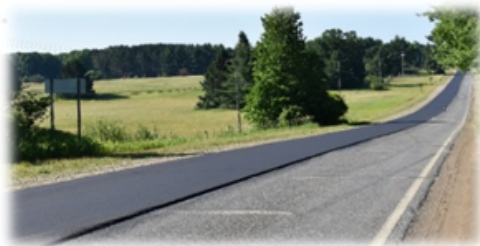
Image: 2018 Clare Avenue Paving
