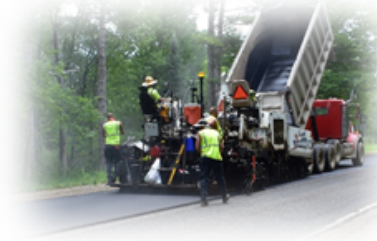
Image: 2018 Clare Avenue Paving
