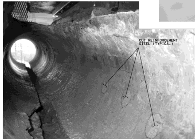
LOCATION OF CUT REINFORCEMENT STEEL
