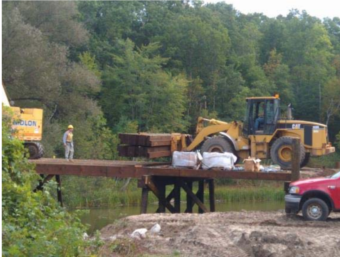
BRIDGE IS STABLE ENOUGH TO LOAD DURING CONSTRUCTION
