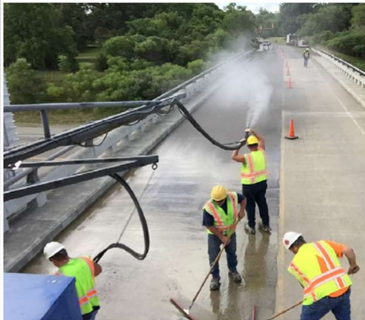
Figure 4. Broadcasting aggregate on sealer.
