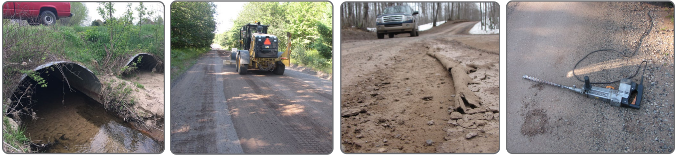
Figure 2: Drainage, shape, material quality, and material thickness are some key considerations when constructing unpaved roads.
