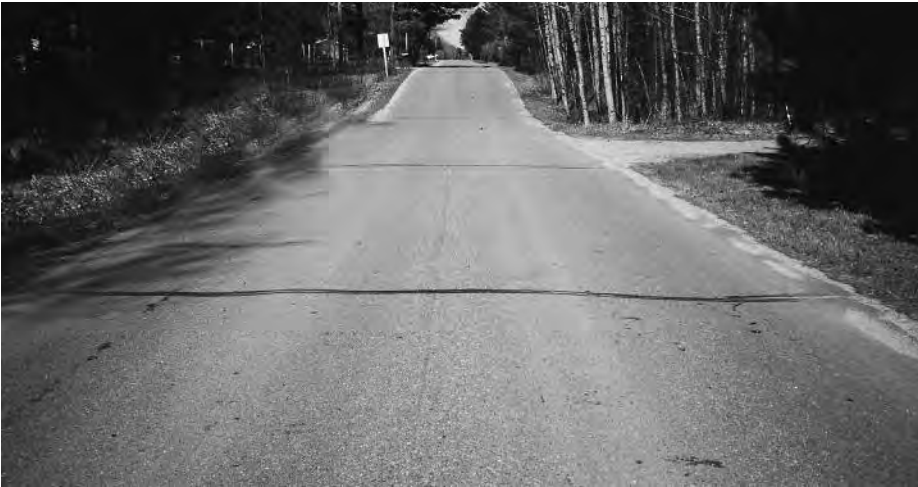
▼ Widely spaced, well-sealed cracks.
