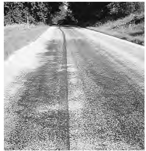
▼ Moderate flushing.
