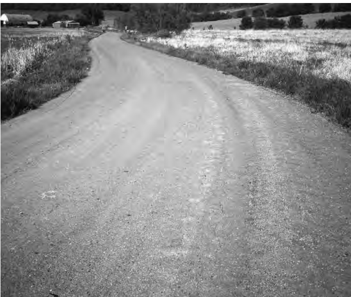
▲ New cold mix surface.
