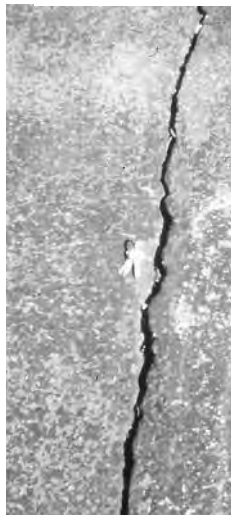
▼ Open crack, 1/2" wide; adjoining pavement sound.
