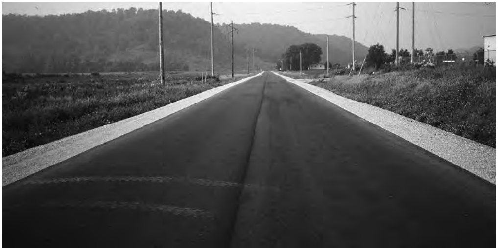
▶ RATING 9 Recent overlay, rural.
