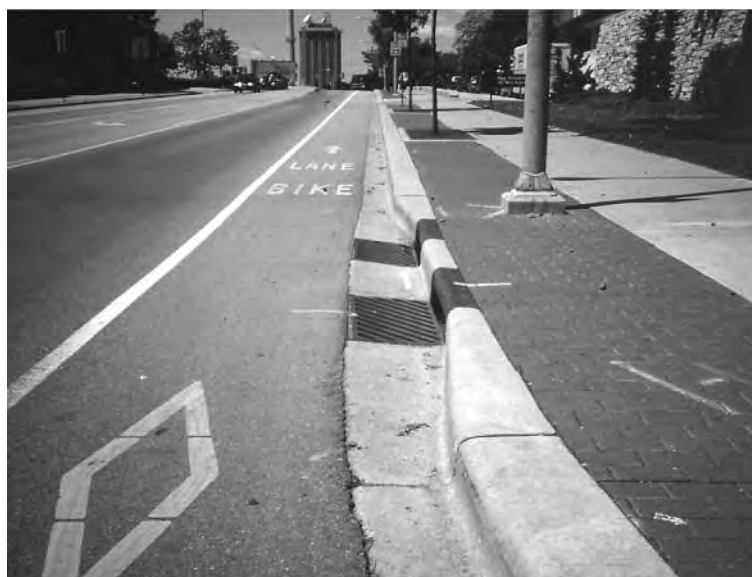
Urban drainage. RATING: Excellent
