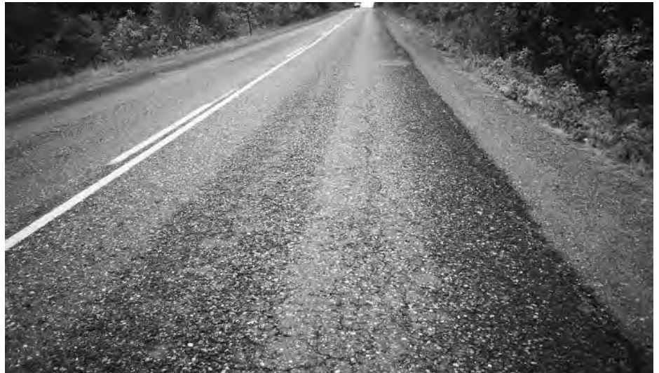
► Moderate to severe raveling in wheel paths.
