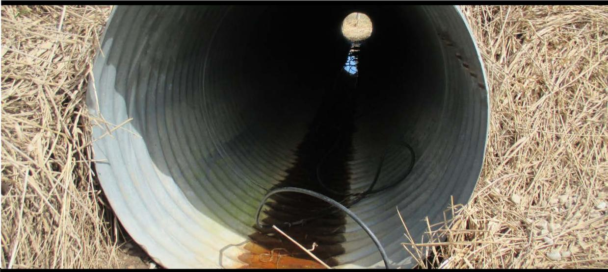
*Figure 10 Corrugated metal barrels distresses like abrasion or corrosion may only apply to a small portion of the culvert's surface area. However, if even a few inches of a culvert's bottom along the entire length of the culvert barrel has been completely abraded or corroded, that abrasion or corrosion can lead to a culvert failure. The severity, the total area affected, and the location of the distress should be considered during culvert assessment.*
