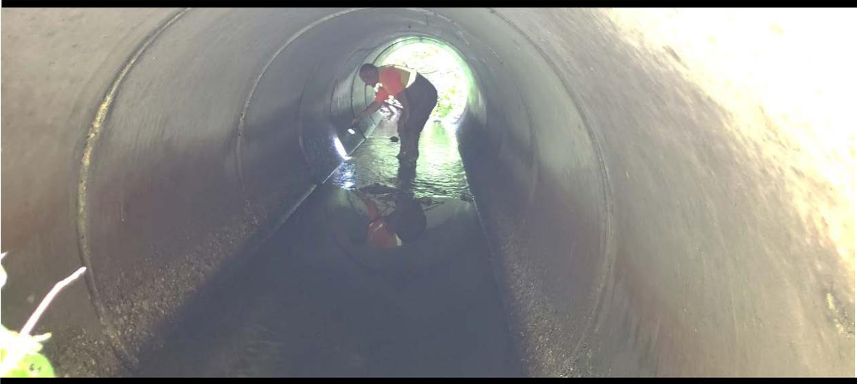
*Figure 9 Concrete barrels should be checked for abrasion along the waterline as well as for signs of infiltration or exfiltration around joints. Performing visual inspections and checking for hollow sounds near joints can help to identify voids that may form as soil around the culvert is carried away. (Photo: Lake County Road Commission)*
