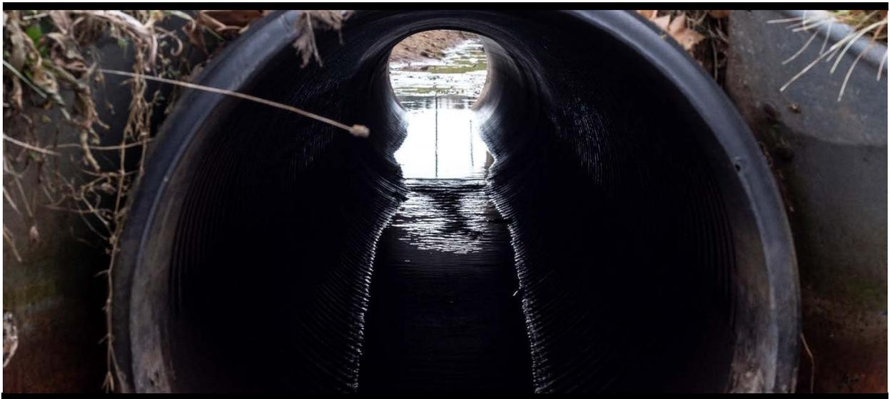
*Figure 8 Plastic barrels may show signs of deformation such as sags, humps, or changes to the barrel's cross section. These changes can sometimes be observed by looking for irregularities in the way that water is flowing through the culvert.*
