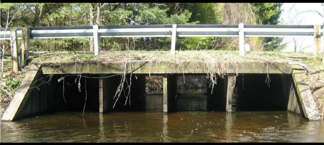
Figure 12 Timber barrel culverts are often in the form of a multi-cell culvert. The width of each cell can be recorded in addition to the total span of the culvert. (Photo: Fleis & Vandenbrink Engineering)
