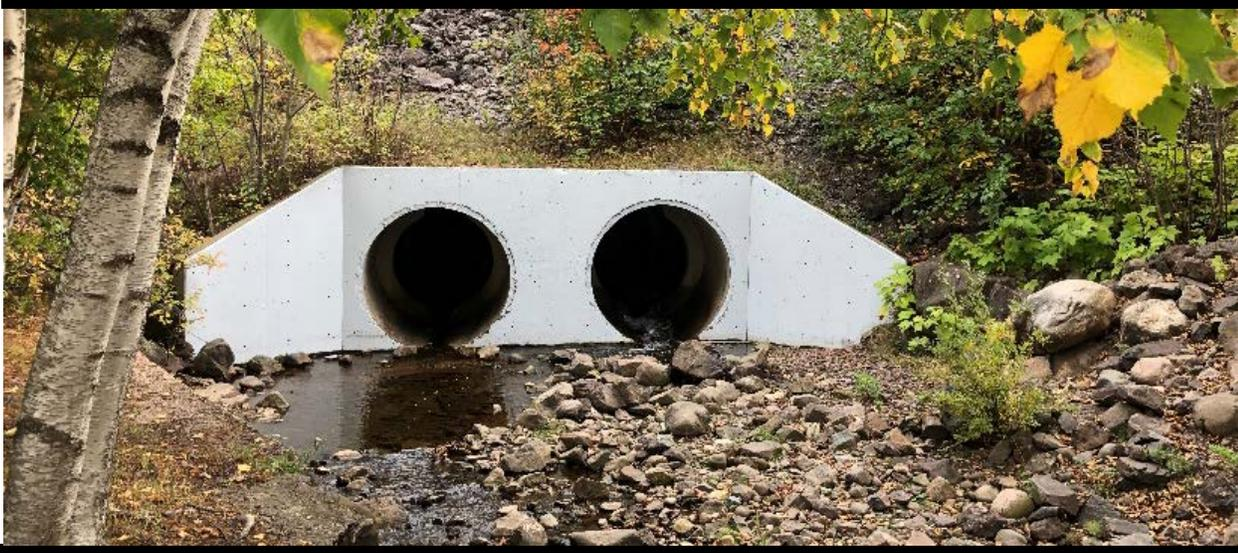
*Figure 7 End treatments should be inspected in relation to the surrounding vicinity. In this photo, the end treatment appears to be in good condition, but there are signs of ponding and movement of stream protection (more riprap in front of one barrel than the other).*
