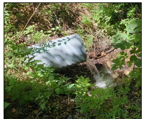
*Figure 6 Erosion can result in a perched culvert barrel where water cascades from the outlet. This falling water can result in further erosion and eventually undermine the culvert barrel to the point that it bends or rotates downward and impedes stream flow.*
