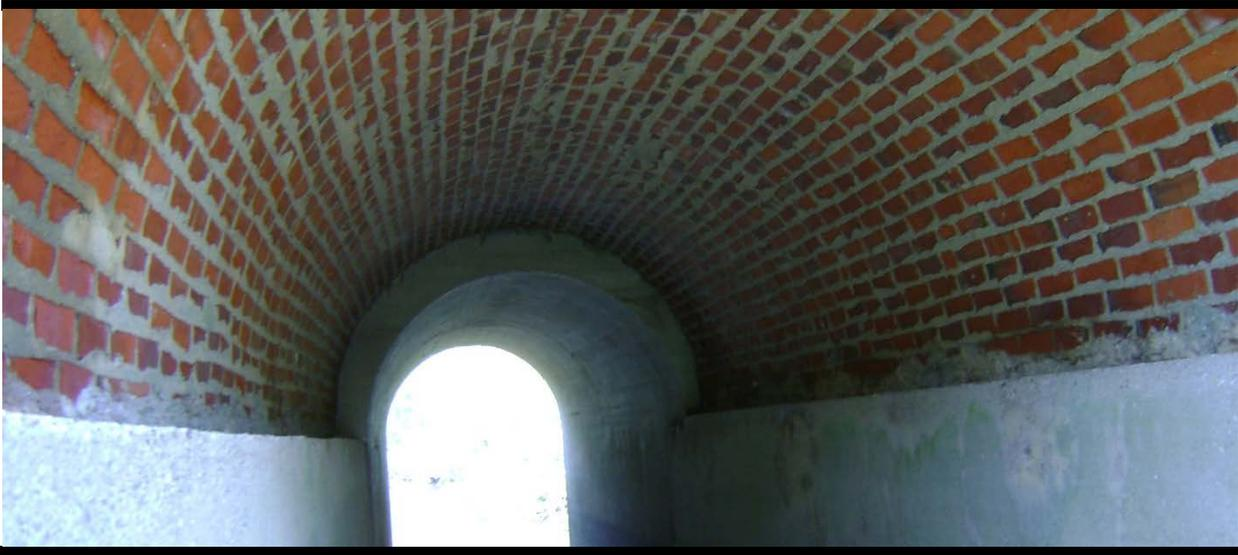
*Figure 11 Masonry barrels are checked for movement of masonry units, mortar, and efflorescence. Note that new mortar or repairs may appear different from original construction. (Photo: St. Clair County Road Commission)*
